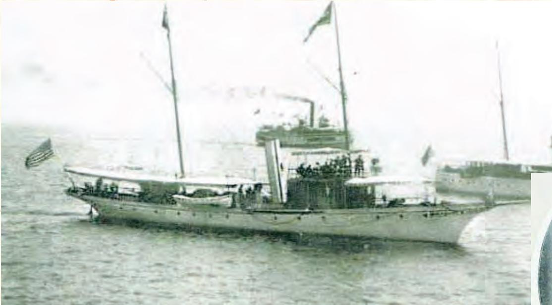
The Enquirer was launched from the yard of the Union Dry Dock Company in 1896, costing some \$75,000. The vessel measured 123 feet, with a beam of 17 1/2 feet and 28 by 16.
